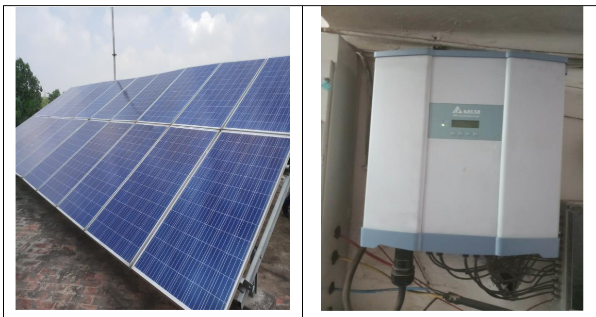
Figure 3.1 Solar Plant 30 KWp and Inverter System
