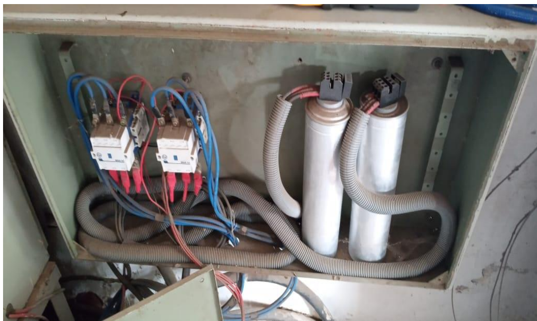
Figure 2.4: - Capacitor bank in Electrical room
