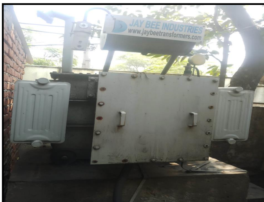
Figure 2.1: - 11 KV Feeder and 160 KVA TR
