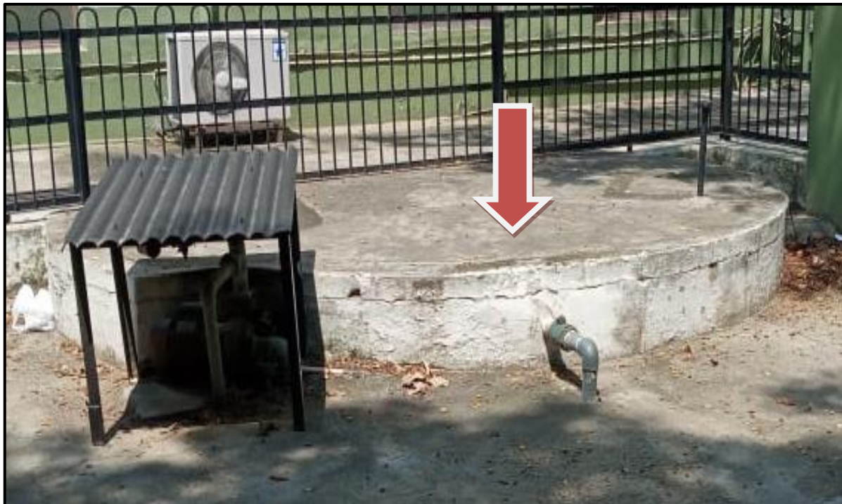
Fig :- 2.2 Water Storage Tank and capacity of College Campus
